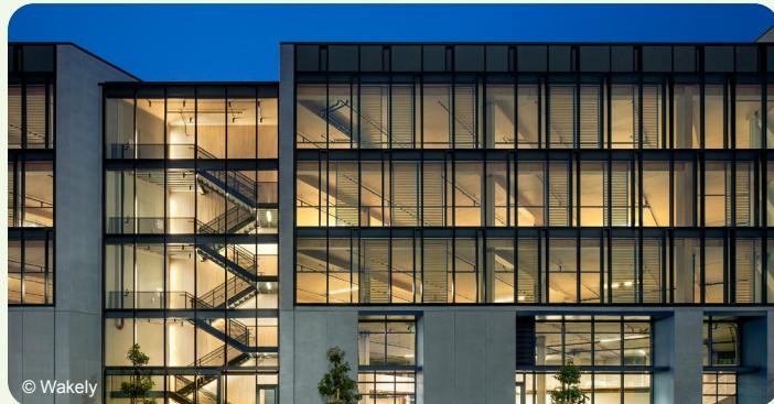
The upper floors were constructed with a CLT slab and glulam post and beam structure. For noise dampening, the CLT floors were topped by concrete with an acoustic mat. The stunning wood elements of 1 De Haro inspired a glass curtain wall that wraps the building, naturally lighting the space and showcasing the material to the outside world.
