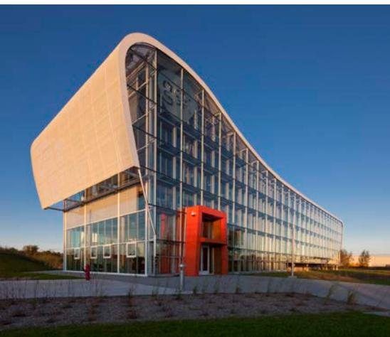
Nordic Structure's FSC-certified engineered timbers in new GlaxoSmithKline offices in Québec.
